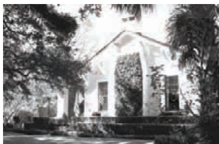
107 Ryan Avenue – Craftsman style bungalow constructed in 1921 for Alan C. Denby.
