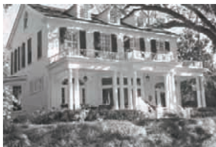
2254 De Leon Avenue – 1908 Georgian Revival style home designed by architect George B. Rogers.
